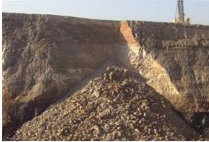
Fig.2. Photo of rib spalling failure at high rock bench
