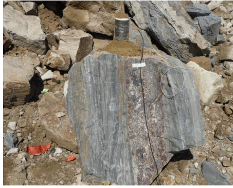
Fig. 15. Placement of the linear shaped charge structure.
