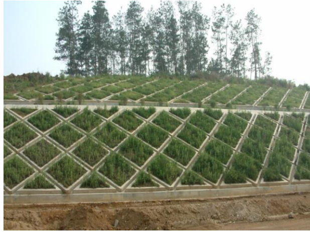
Fig.2.Effect drawing of frame beam slope protection
