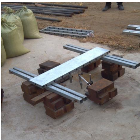
Figure 1: 0.2\text{m} \times 1\text{m} formwork diagram diagram of (after the dial indicator is adjusted to zero )
