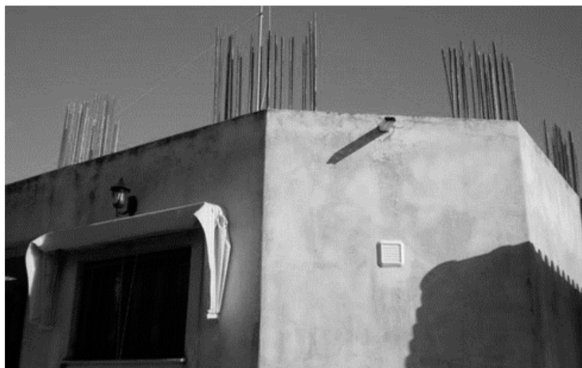
Fig.1. The existing structure
