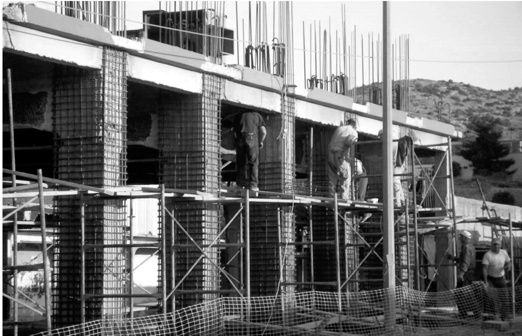
Fig.9. Construction of reinforced concrete jackets
