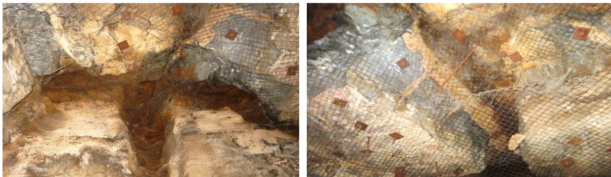
Fig. 2. Solution Cavities of Shale and Dolostone of the H/W Lode
