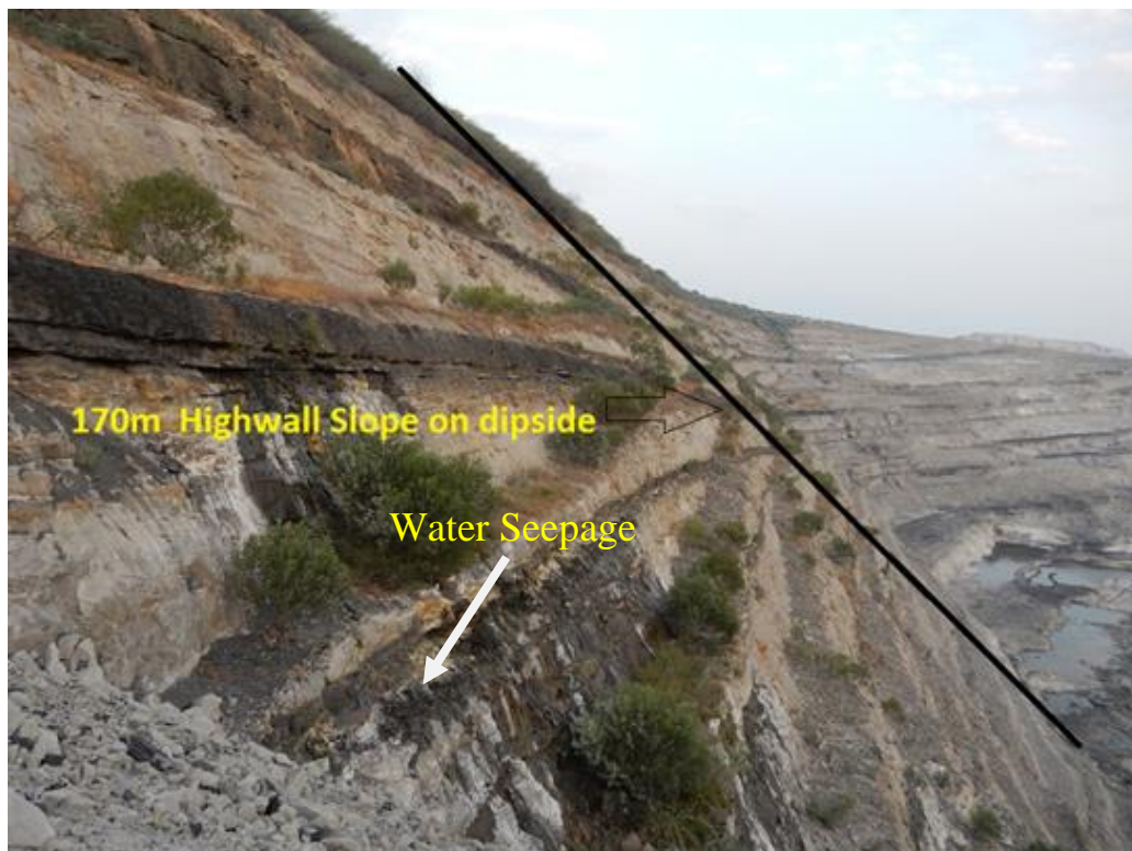
Figure 2.4. Photograph depicting the ultimate of 170m highwall of Medapalli OCP
